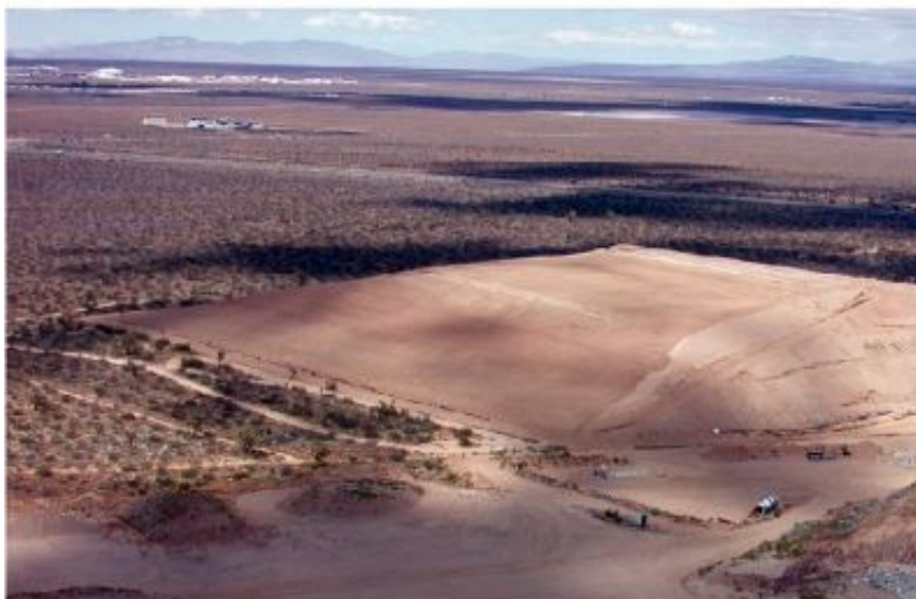
A leach pad on top of an old mine bearing gold ore in the Mojave Desert needed to be brought back to its original condition. See photo on page 34
